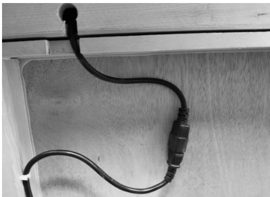
(1) Plug in the connectors of heater cables, make sure the cables not pinched between ceiling panel and other panels.
